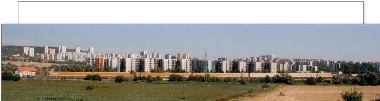
The hugest anti-noise barrier (the height 7.5 m and length nearly 2 km) in the Czech Republic, protecting 15,000 inhabitants of Brno – Bohunice.
